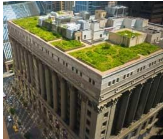
Figure 4: An example of a green roof on top of Chicago City Hall. [18]
